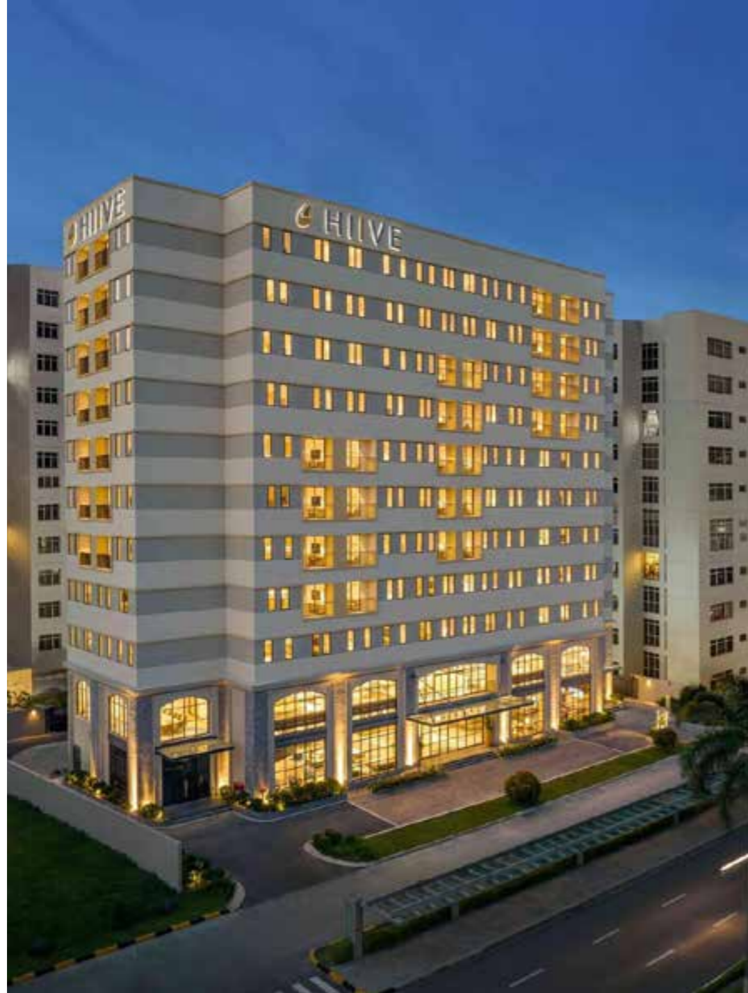
Main view from the street
